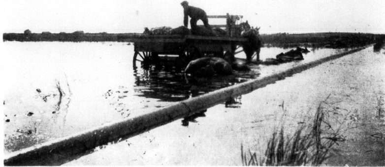
Floating Pipe Through Slough
