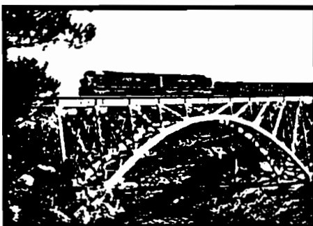
Ore train crossing the Spring Creek Bridge on the journey to Dampier.
