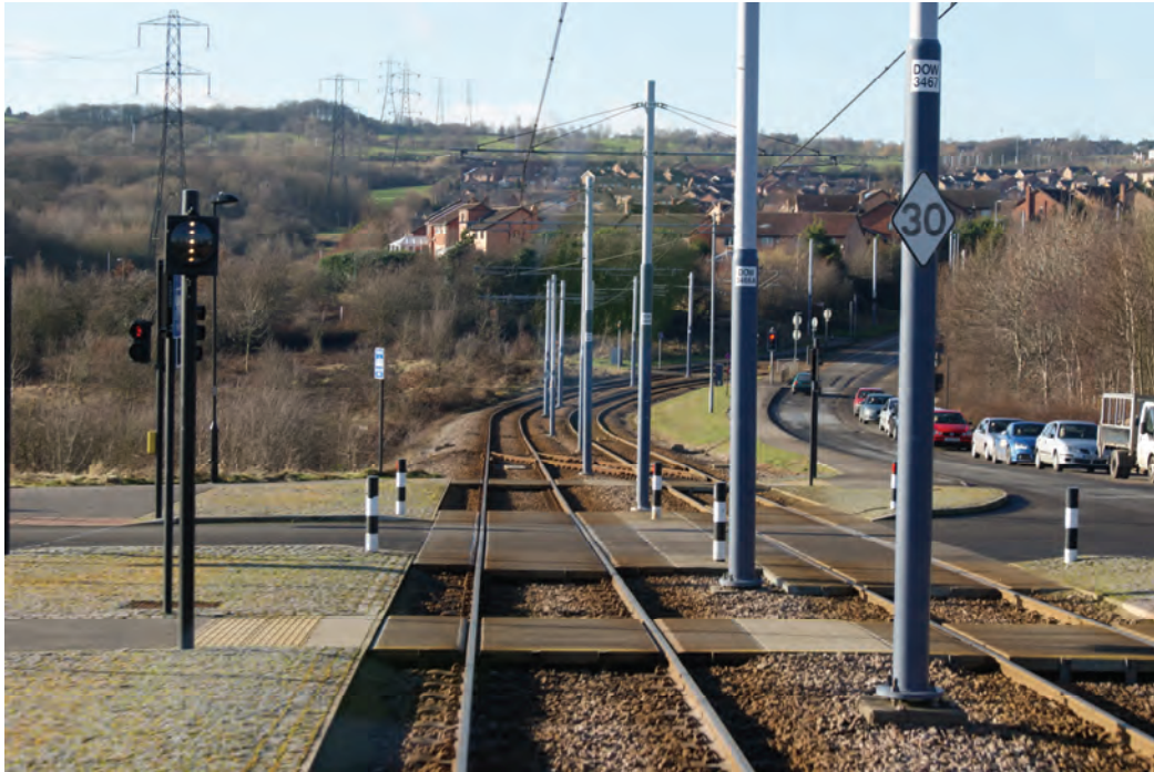
Pedestrian and highway crossings on the tramway in Sheffield, shown from the perspective of the tram driver. Note the tramway signals and ordinary traffic lights.
